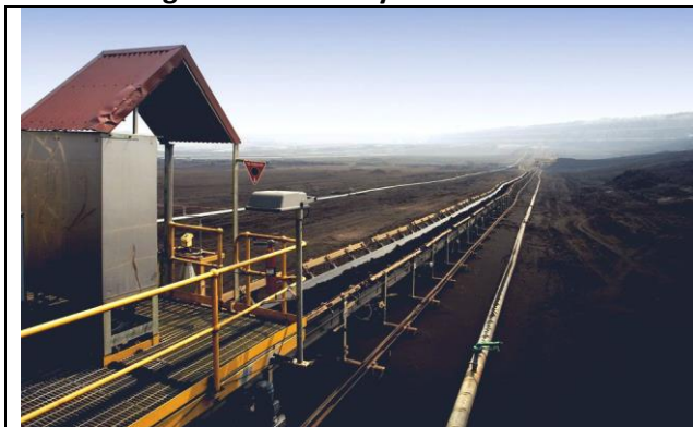
Source: www.thiess.com/projects/yallourn-mine-alliance (Enclosed Conveyor is the intent of MRV)
